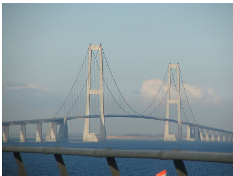
Figura 30 – Ponte Great Belt Bridge
