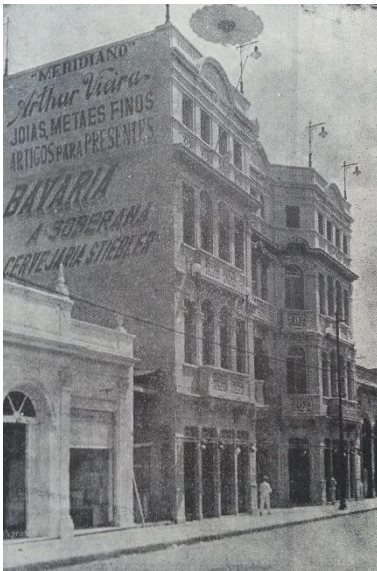
Figura 13: Galeria Pio X, Rua Halfeld, (1930-40?).
